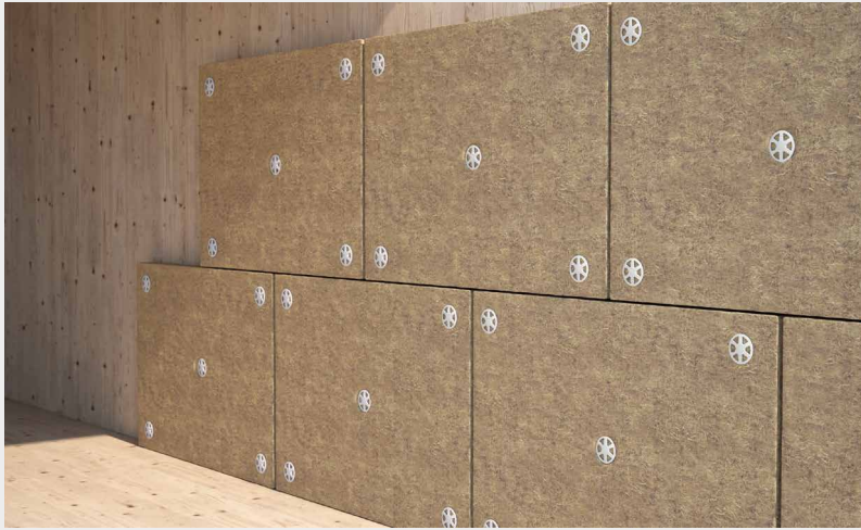
Wall insulation boards fastening with THERMOWASHER and HBS 8 mm diameter.
